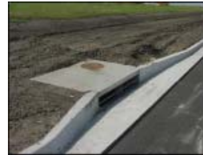
Curb and gutter system
