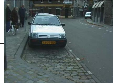
permeable paving on sidewalk and on-street parking
