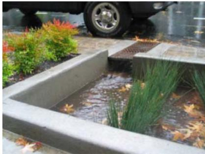
The stormwater swale by the on-street parking
