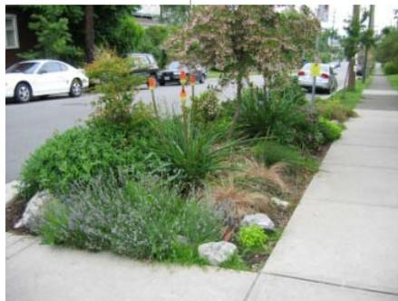
Using the bump-out to be the landscaping infiltration basin to filtrate and infiltrate stromwater runoff
