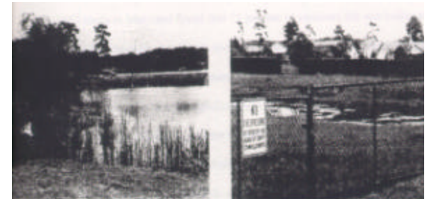
Wet and dry detention basins
