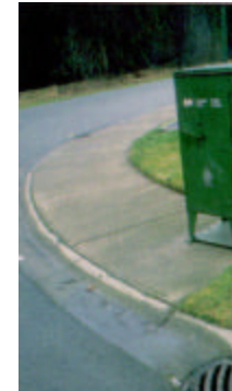
Conventional curb and gutter system
